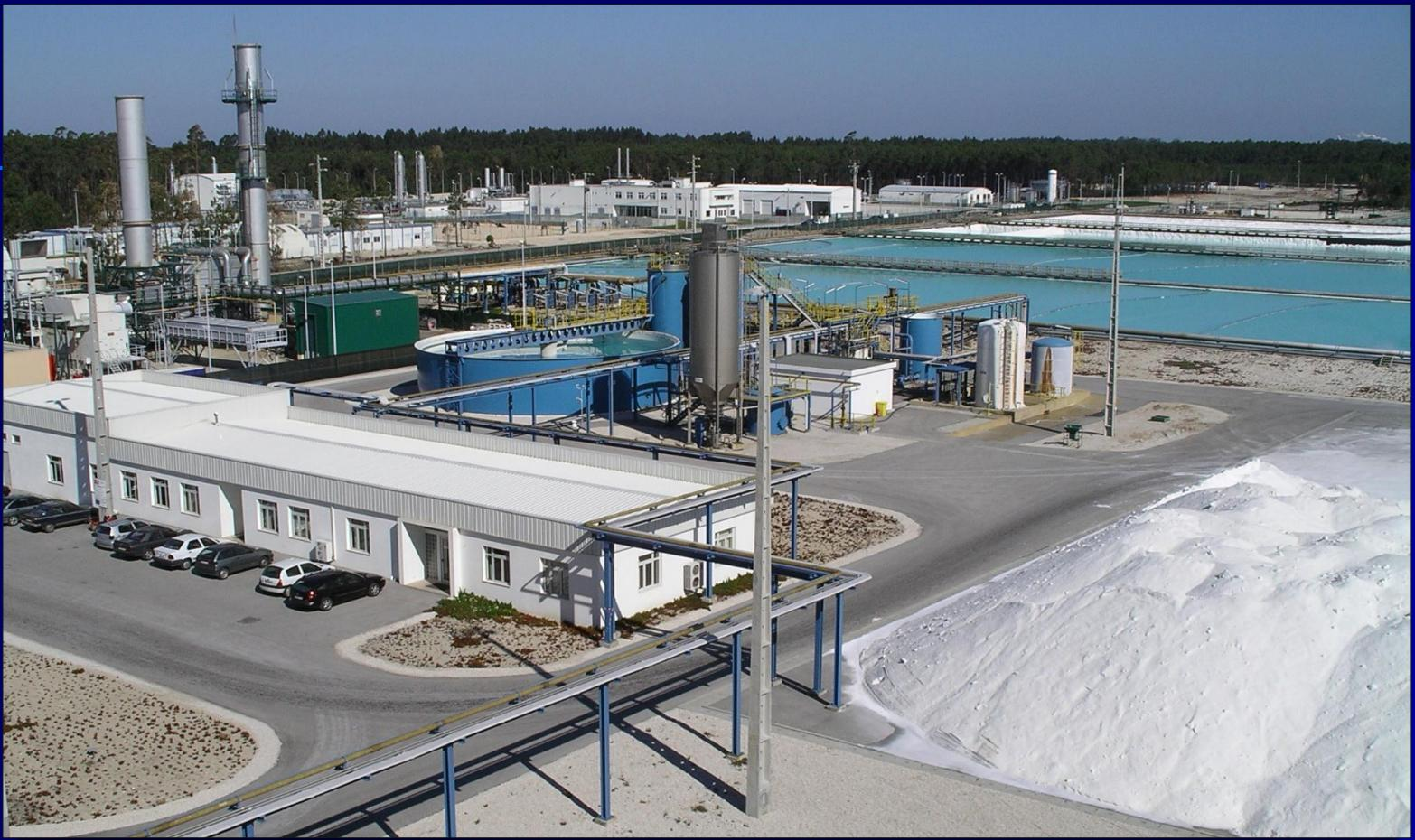
**Solution mining for natural gas storage, co-generation, brine purification, salt crystallisation and refining plant in Portugal**
