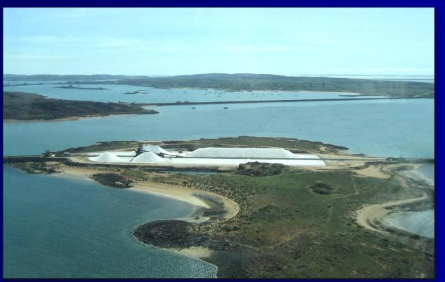
The two Dampier original intermediate stockpiles are now used to dry the salt washed in a new washing plant. They are 400 m long and 55 m wide. They can hold up to 500'000 t. In 2009 the pictured stock was estimated at about 170'000 t or 36% of design capacity.
