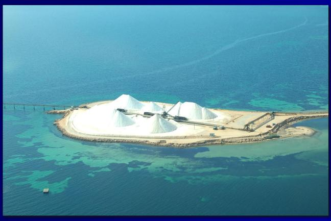
The Shark Bay stockpiles are 200m long and 60m wide. Their design capacity is 250'000 t. In 2009 they were less than half full.
